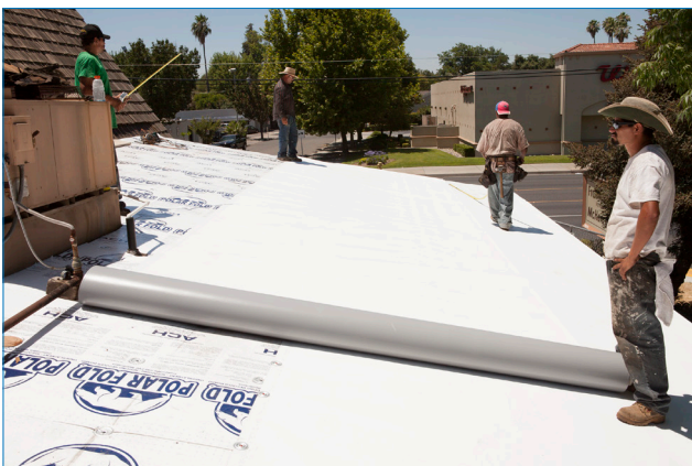
TPO roof installation
